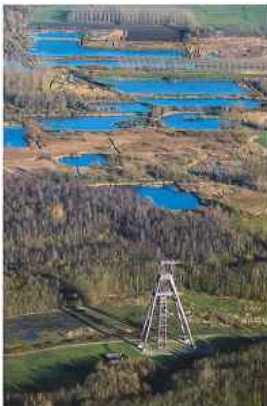
Chevalement Chabaud-Latour, Condé-sur-l'Escaut (Nord)-©-Philippe Fruitier - Altimages
